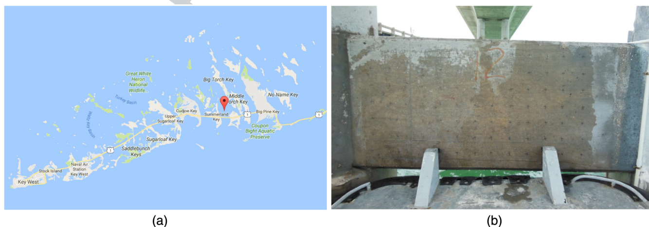
FIGURE 1. Niles Channel Bridge location and the investigated strut (0.9 m × 1.8 m). (a) Google map and (b) photograph of the strut.
